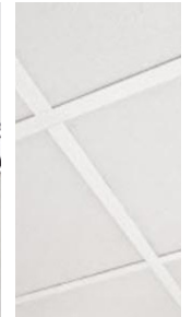
Suspended Ceiling Grid
